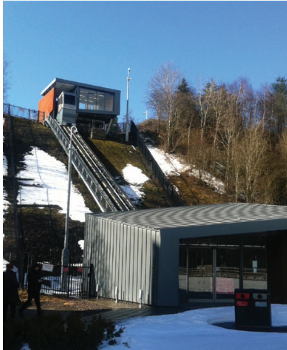
Figure 34, Mechanical lift at Ebbw Vale
