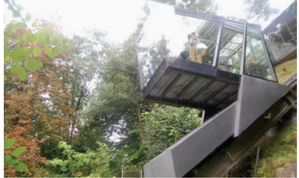
Figure 9, Example of contemporary inclined lift at Lubiana
