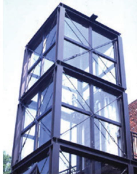
Figure 8, Example of stand-alone external lift tower
