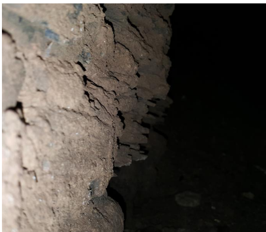
Figure 10 The jamb of the second firebox.
