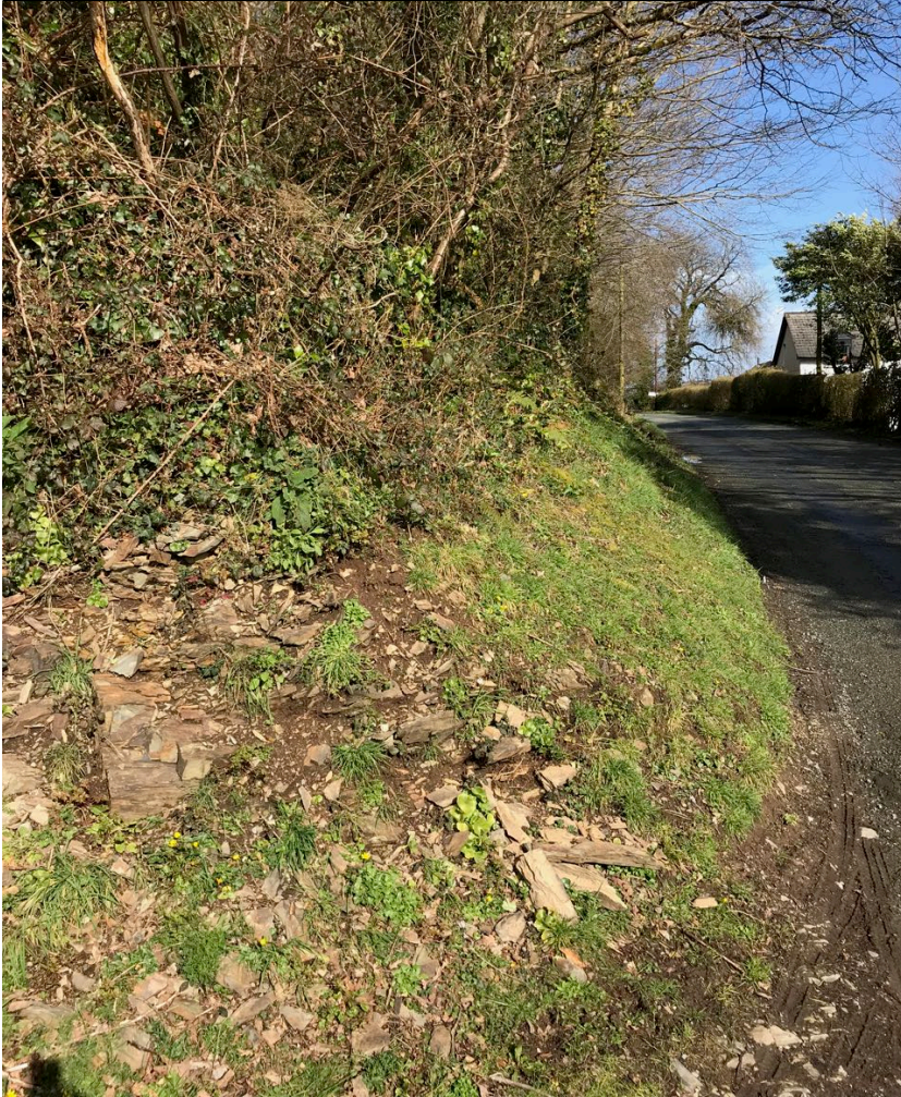
Figure 17: Embankment at junction opposite Glanteifi
