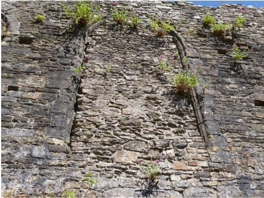
Fig 7 Blocked upper window of east range showing late C13 mouldings
